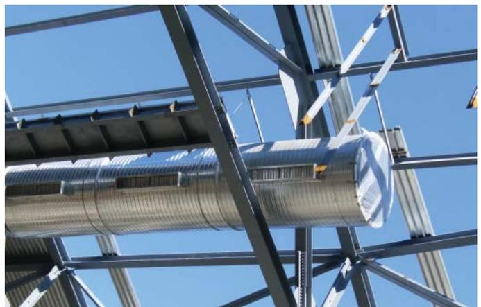
double-wall spiral duct as well as interior duct for the perimeter spaces of the arena. The manufacturer customized rectangular saddle taps to fit inside the round duct. These taps housed the large air diffusers required to direct air all the way to floor level of the arena. The
