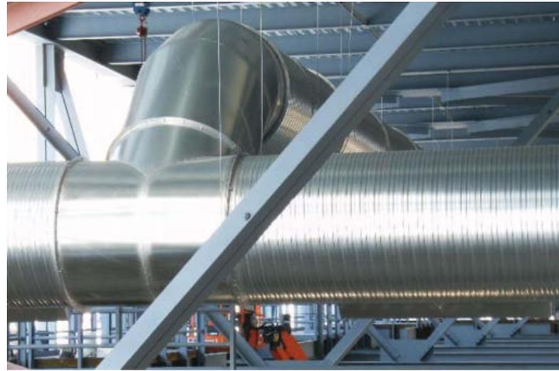
sections of duct were completely pre-fabricated with special flanges located at optimum intervals. The saddle taps were welded per the engineering firm's design. Volume dampers and accessories were also factory installed.
