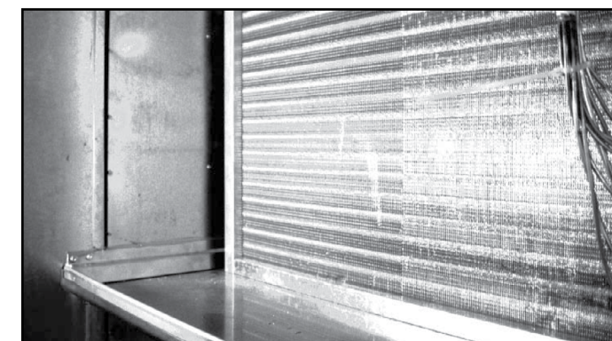
FIGURE 28. Cooling coils should be checked for leaks during operation.
