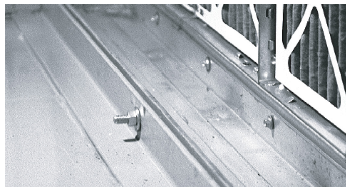
FIGURE 9. Field joint located at floor.
