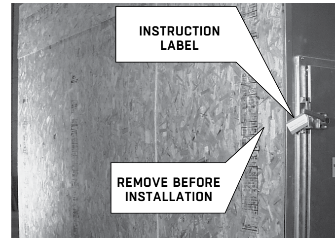
FIGURE 4. Module sides which are to be joined at time of installation are covered with plywood and/or plastic sheets for protection during transport. Throughout the unit you will find instruction labels indicating which steps MUST be performed for proper installation.
