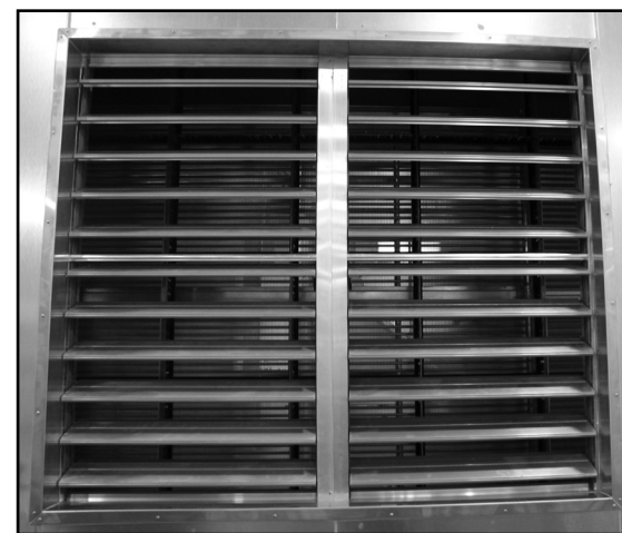
FIGURE 11. Be sure that damper blades open and close properly and have sufficient rotation clearance.
