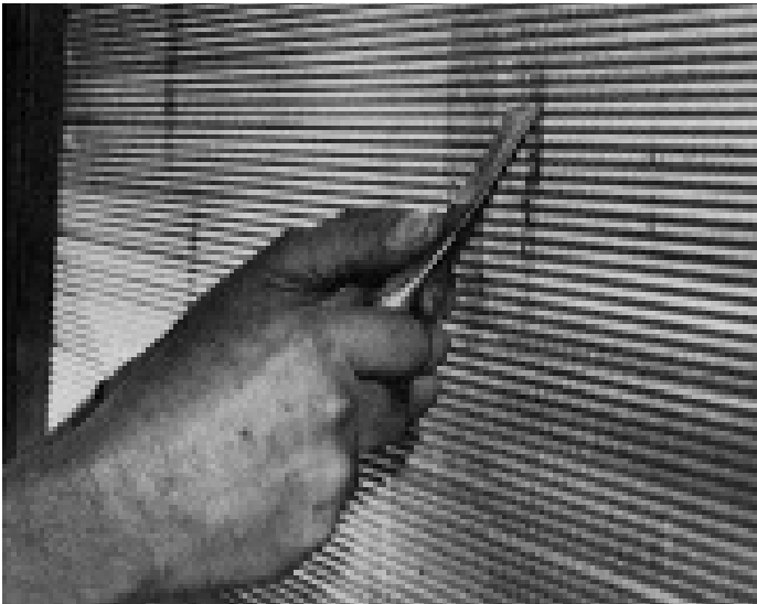
FIGURE 44. A fin comb may be used to remove matter entangled in fins, as well as to straighten fins. But normally flushing coils with water under normal pressure will remove most matter.
