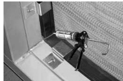
FIGURE 23. On the weather side of the wheel where face seal meets perimeter seal at both ends.
