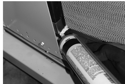
FIGURE 22. Purge seal where it meets perimeter seal.
