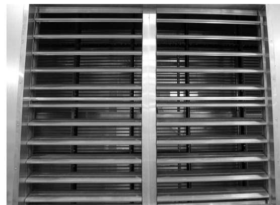
FIGURE 40. Be sure that damper blades open and close properly and have sufficient rotation clearance.
