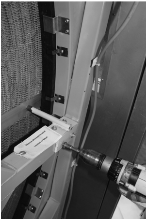
FIGURE 13. Shipping restraint for flat rim wheel.
