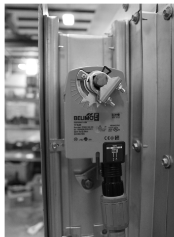
FIGURE 41. Damper actuator
