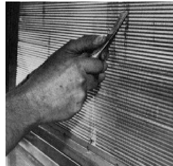
FIGURE 24. A fin comb may be used to remove matter entangled in fins, as well as to straighten fins. But normally, flushing coils with water under normal pressure will remove most matter.
