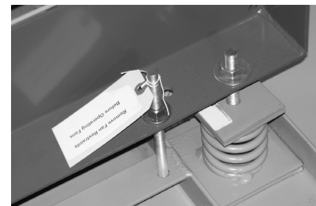
FIGURE 17. Two restraints at the base of the rear of the fan.
