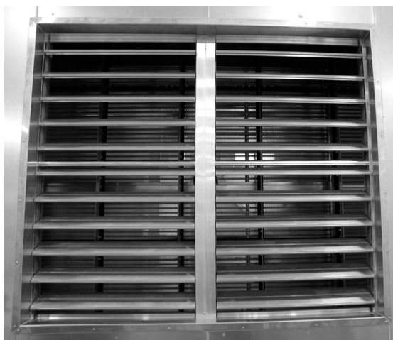
FIGURE 20. Be sure that damper blades open and close properly and have sufficient rotation clearance.
