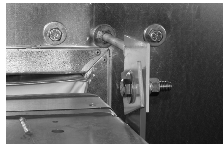
FIGURE 15. Two restraints at the top of the fan bolting the fan to the wall.
