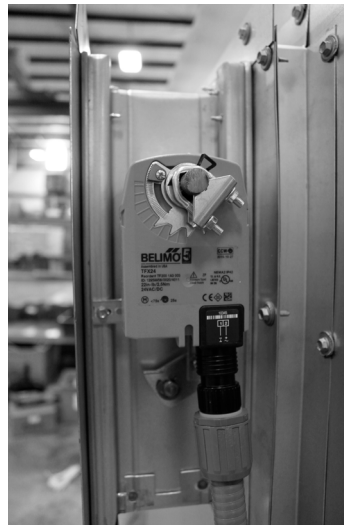
FIGURE 21. Damper actuator
