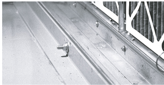
FIGURE 7. Field joint located at floor.
