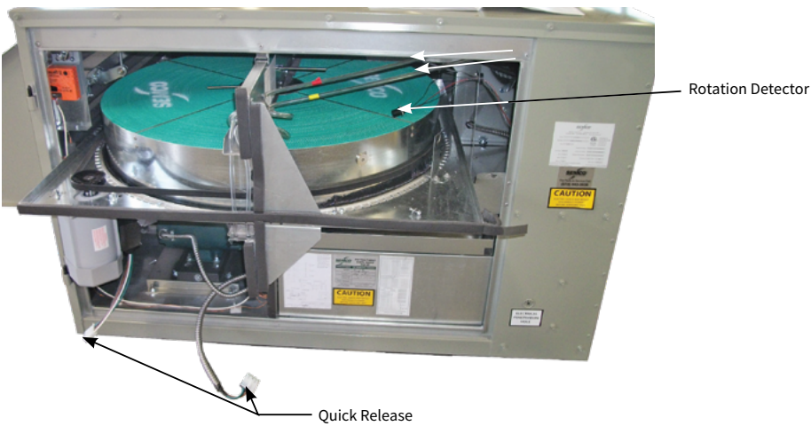
FIGURE 19. Prior to sliding out the wheel cassette, the wheel motor quick releases, and the rotation detector sensor must be disconnected.
