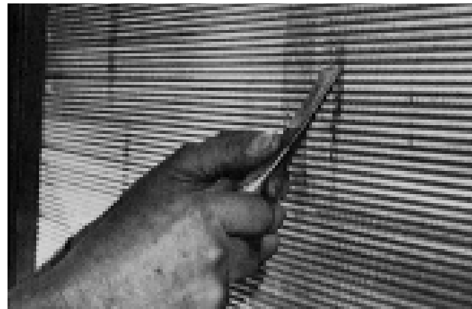
FIGURE 28. A fin comb may be used to remove matter entangled in fins, as well as to straighten fins. But normally flushing coils with water under normal pressure will remove most matter.
