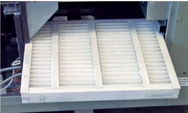
FIGURE 14. Replacing return air filters.
