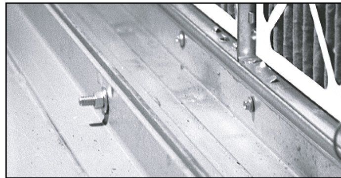
FIGURE 7. Field joint located at floor.
