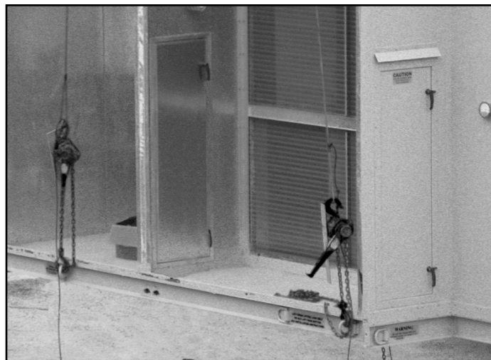
FIGURE 1. Lift modules only with lugs located at the base of each module. Do not use a forklift. NOTE: Chain hoists used to level unit.
