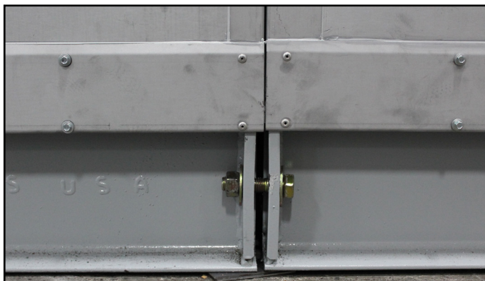
FIGURE 5. Field joint located on base. Use only these bolts to pull the modules together.
