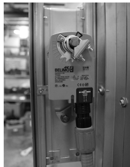
FIGURE 28. Damper actuator.
