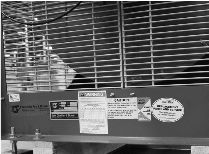
FIGURE 33. All fans installed in FläktGroup SEMCO systems are labeled with lubrication instructions that should be followed. On smaller fans the label can be found on the fan frame.
