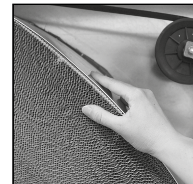
FIGURE 18. Rotate the rotor at least three turns in the direction indicated by the rotation arrow.
