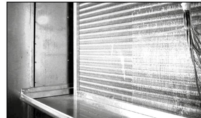
FIGURE 29. Cooling coils should be checked for leaks during operation.
